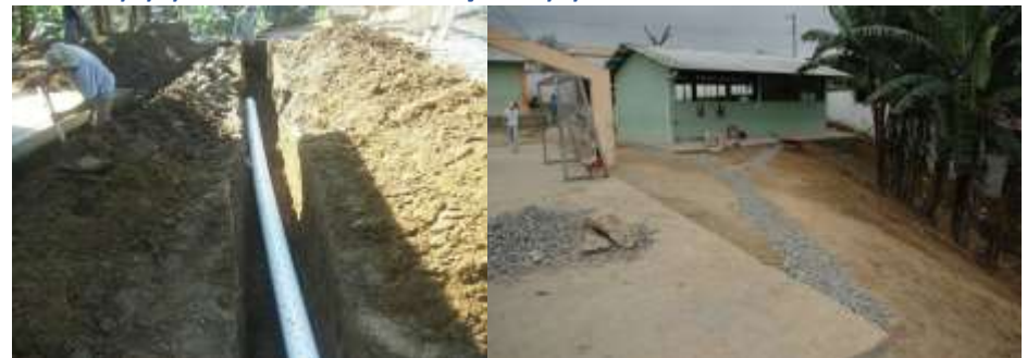
Underground perforated PVC pipes and aggregate filling (Credits: A. Petrone)
