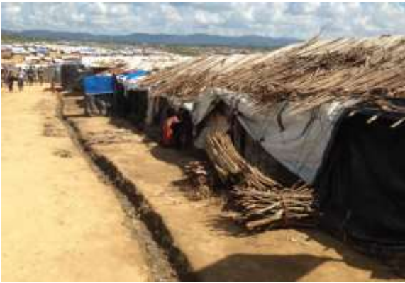
Lined ditches with bamboo mats and cement lining
